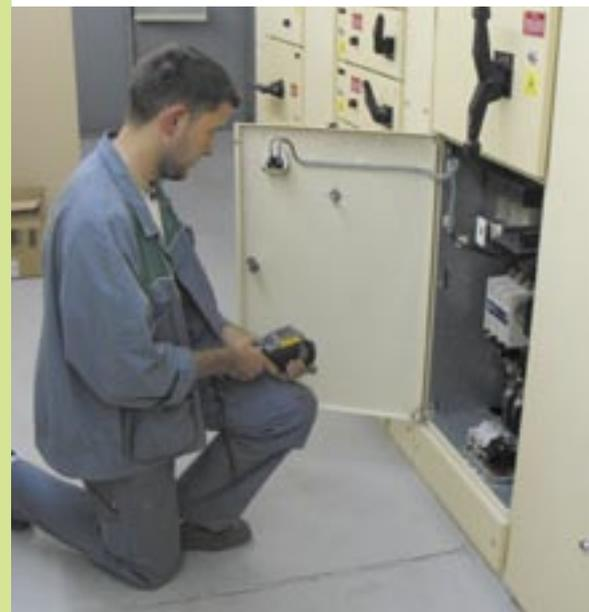
After Diagtech has done the inspections, and we have carried out the necessary repairs, we use the infrared camera to see if the problem is really solved."
